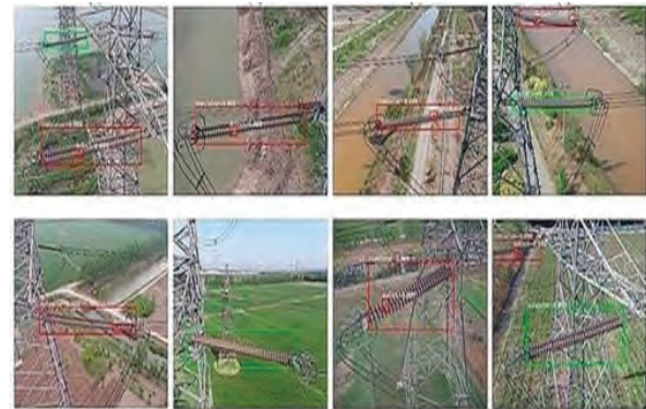
Fig. 5: Insulator defect detection
