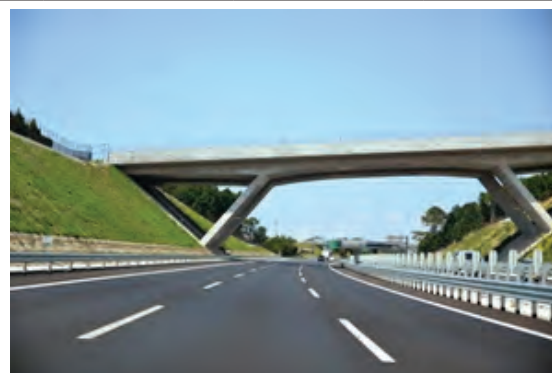
Fig. 2. A1 renewal project [17]
